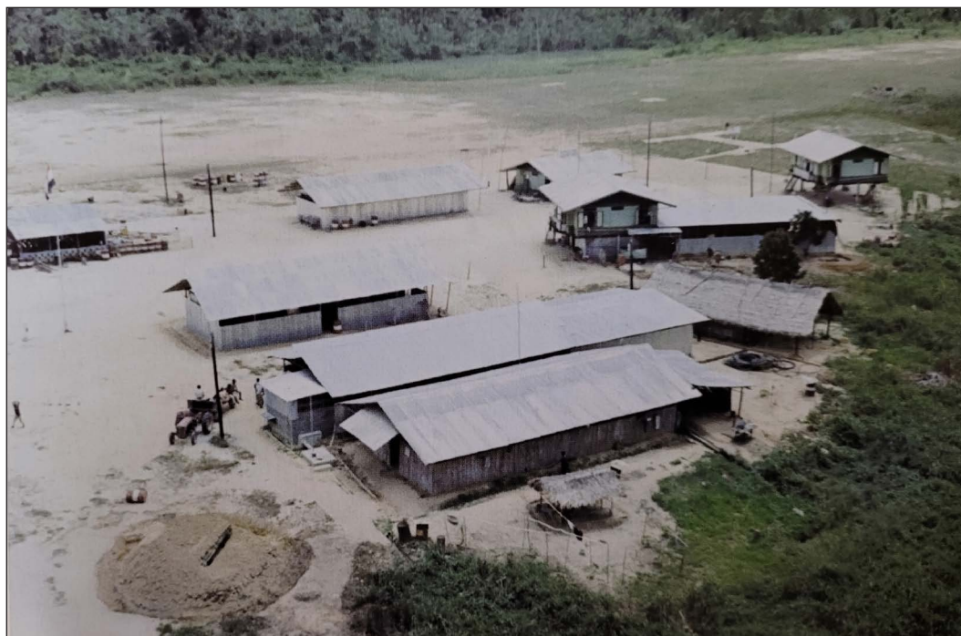
The TRIS outpost at the Coeroeni. It was built in the late 1960s in order to support DEFPOL and to monitor Guyanese activity in the area. (NIMH Collection/W.M.M. Calting-Houwing)
