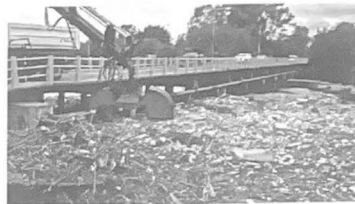
Argentina. An $80m loan approved by the EIB to upgrade the Partido Escobar sewer network and wastewater treatment plant will improve access to sanitation services for more than 24,000 residents
