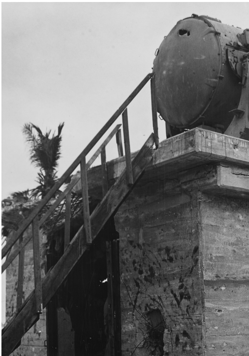
A Japanese blockhouse on Betio Island, November 1943. Admiral Chester W. Nimitz, CINCPAC, and a party of Navy and Marine Corps officers inspected this and other installations on Betio after the island's seizure. Recognition of the ineffectiveness of American naval gunfire against many enemy fortifications during the Tarawa invasion initiated a cycle of rapid improvement in the planning, training, and application of naval gunfire support in the Pacific. (NHHHC, NH 62567)
