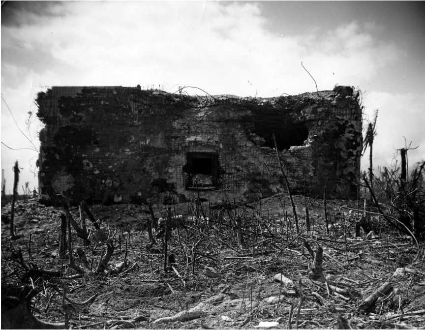
Destroyed blockhouse on Roi-Namur Island, February 1944. The contrast with naval gunfire effects achieved at Betio only two months before is obvious. (NHHC, S-065)
