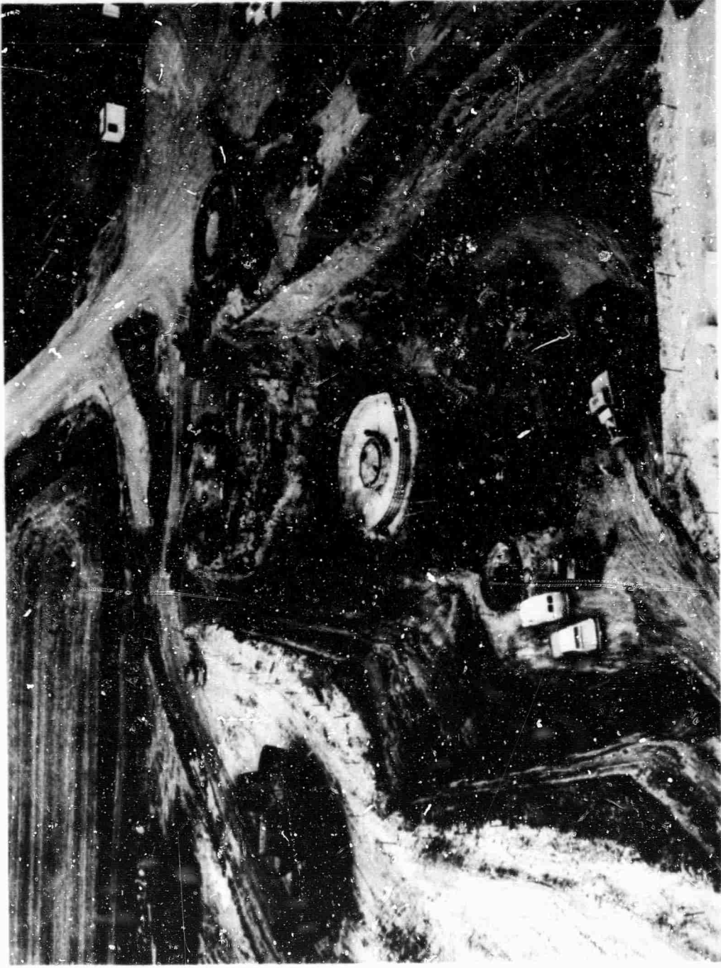
Fig. 9. Minuteman excavation; wet base-level due to seepage from toe of slope
