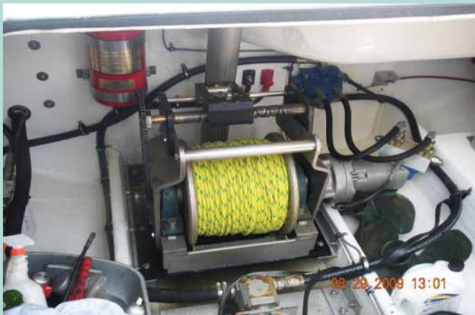
The winch, hydraulic system, hoses, and towline onboard the vessel.
